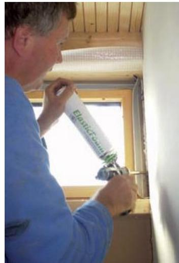
Extrusion de la mousse expansive
