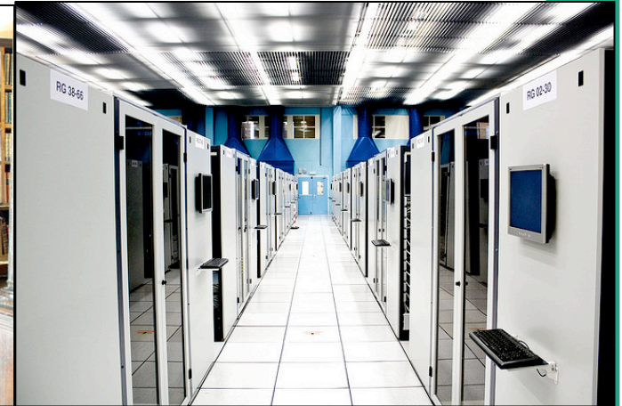
Server room at CERN by Torkild Retvedt is CC-BY SA 2.0
